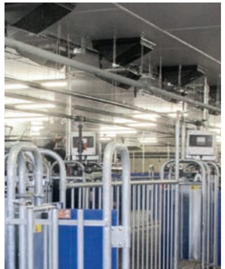
Fin heater as a full-space heating system – ideal in combination with ceiling inlets
