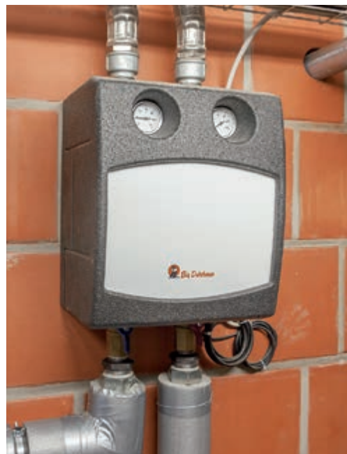
Three-way heating control
